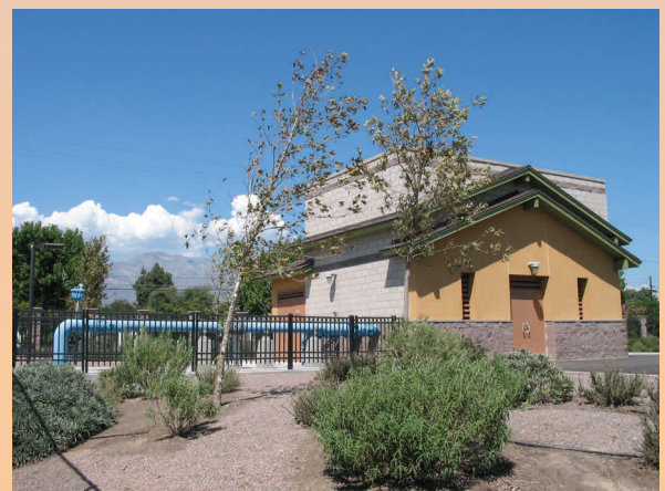
ASR Well 30 Pump House
